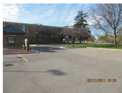
6 4 PHOTO 3 LOOKING SW. @ NORTHERN ENTRANCE/DRIVEWAY TO CITY HALL SITE. PHOTO TAKEN 11/2/2011, ECT.
