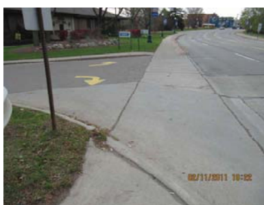
5 4 PHOTO 2 LOOKING SE. @ NORTHERN ENTRANCE/DRIVEWAY TO CITY HALL SITE. PHOTO TAKEN 11/2/2011, ECT.
