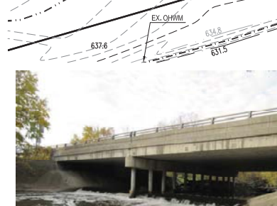
7 PHOTO 7 2 LOOKING E. @ EXISTING EROSION AREA AND LOG JAM. PHOTO TAKEN 11/2/2011, ECT.
